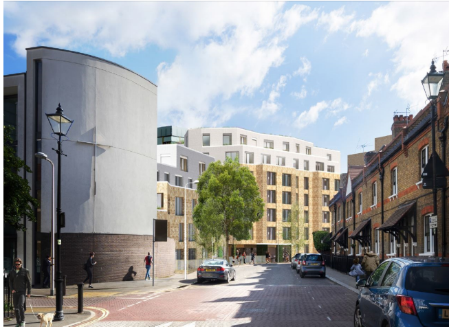
Figure 2: View eastwards along Ufford Street, showing Block A of the hotel in the foreground and Block B behind.
